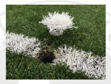
2. Locate and remove the caps for the three support posts at the rear of the goal. These caps are a lighter shade of green and can be removed by pulling on the grass.
