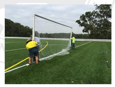
7. Thread the corner and middle net guy ropes through the eyelets at the top of the support posts. Insert the posts into their respective sockets and tie off guy ropes to tighten net.
